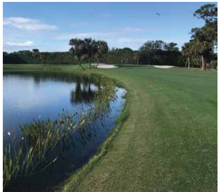
The SOX “Living Shoreline” is sodded over and naturally integrates into existing shoreline. This creates a newly rooted safe, secure shoreline.
